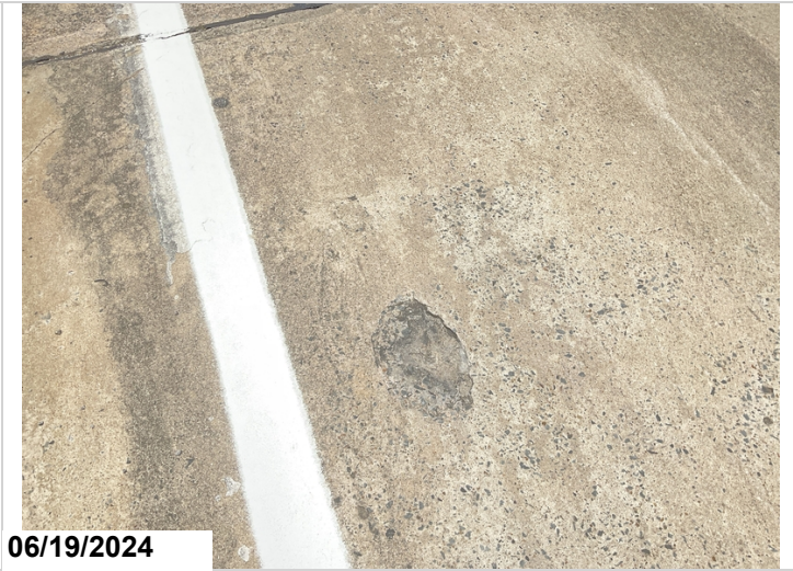
Span 3: Spalling. CS3.
