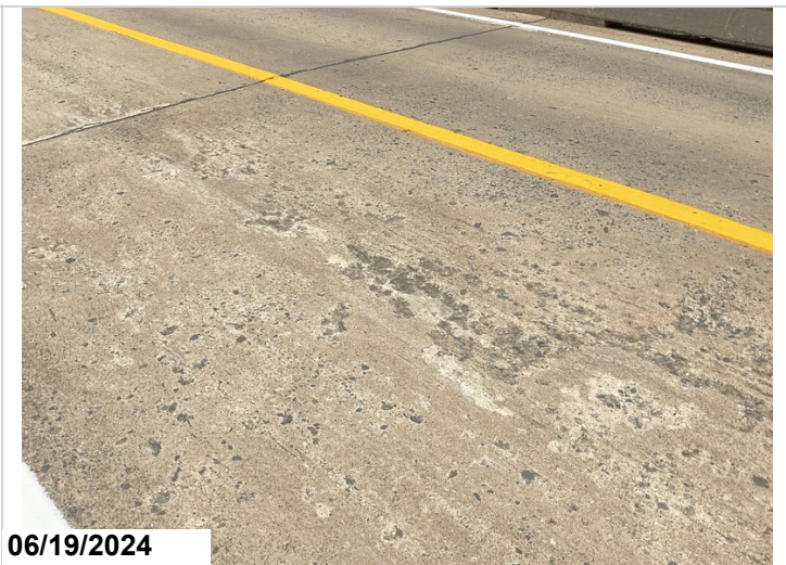
Span 1: Spalling.
