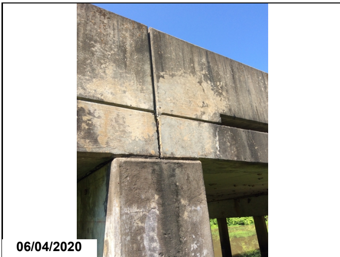
Vertical efflorescent cracks to outside edge of deck at Spans 1, 2, & 3.
