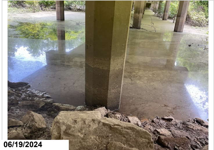
Piles: Minor abrasion throughout the structure. CS2.
