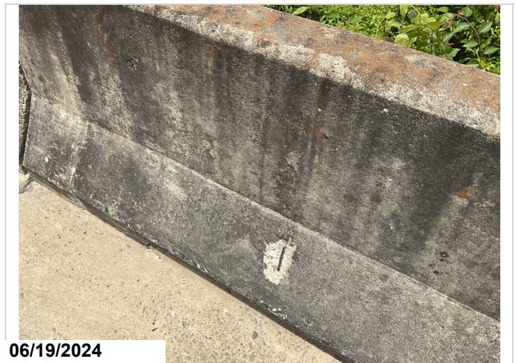
Span 6, Right Bridge Railing: Spalling with exposed reinforcing steel. CS2.
