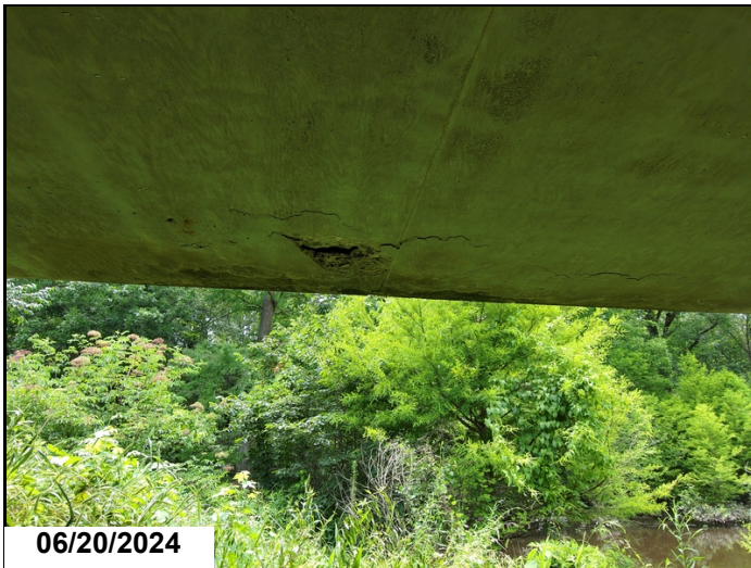
Spall/Areas of delamination to Left & Right edges of soffit at Spans 1-6 & 8-10. Lt side, span 1
