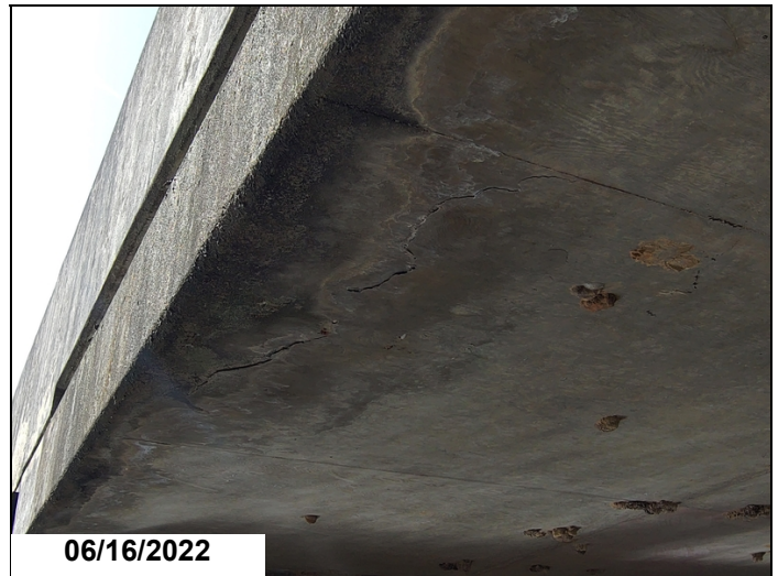
Spall/Areas of delamination to Left & Right edges of soffit at Spans 1-6 & 8-10. Span 3
