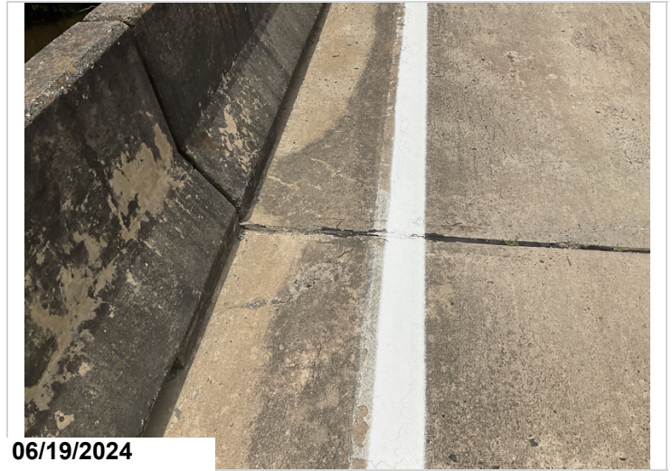
Spans 2 & 3, Left: Diagonal cracking.
