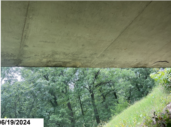
Span 10, Left, Undersurface: 7' of delaminated areas. CS3 2'. CS2 5'.
