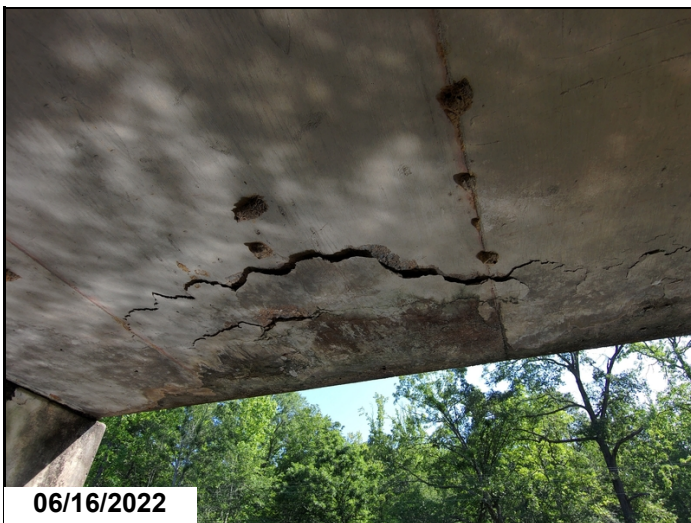
Large delam to rt edge of soffit @ span 2.
