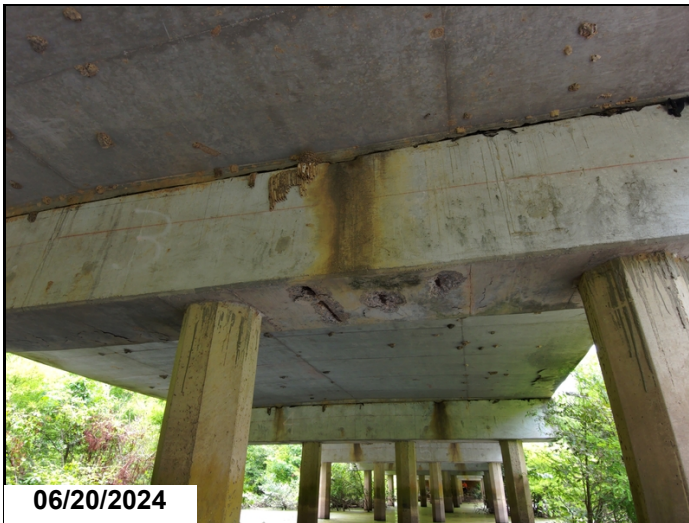
Spalls to cap with rebar exposed at Bents 1, 2, 3, 4, & 5. Bent 3, between piles 3 & 4
